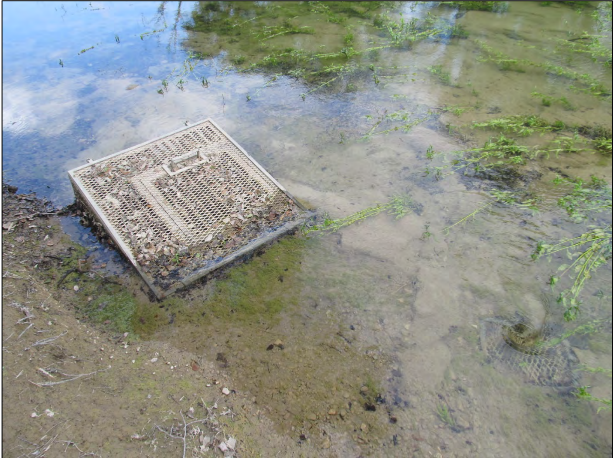
Figure 7-1. Cave gate over Crippled Crawfish Swallet. Note whirlpool in lower right of photograph. Photo by BSEACD.
