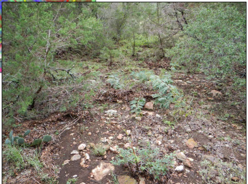
Figure 2. Debris dams formed during October 2013 rains near Flint Ridge Cave. In areas of subtle relief, these dams may re-direct water from one drainage path to another.
