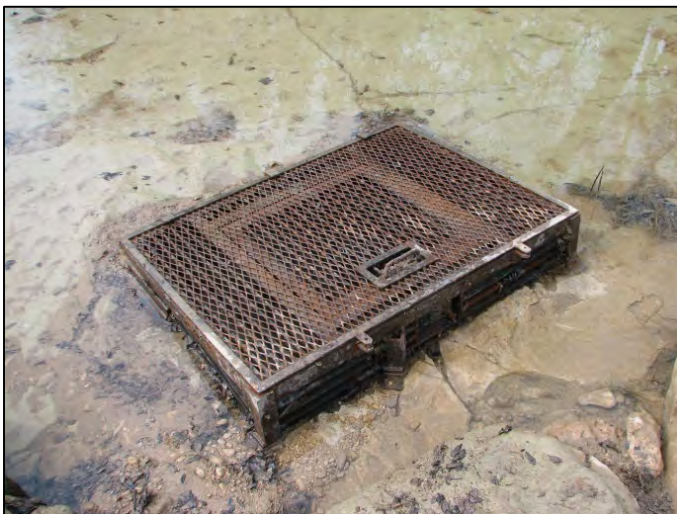
Figure 4. Example of swallet grate with fine debris cover.
